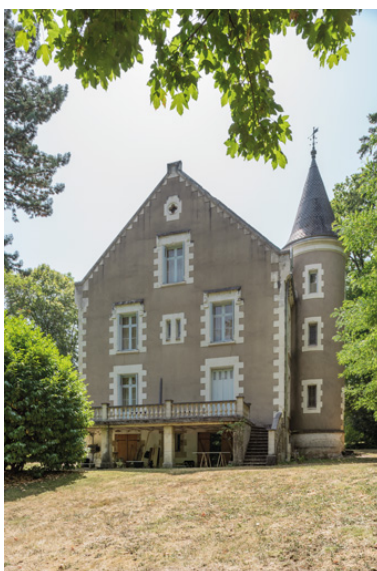
Mur pignon nord-est. Phot. Pierre-Marie Barbe-Richaud IVR26_20195800531NUC4A
