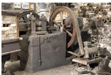
Atelier est. Laminoir. Phot. Jérôme Mongreville IVR43_20087000827NUC2A
