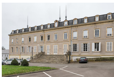
Aile nord, façade. Phot. Pierre-Marie Barbe-Richaud IVR26_20227100049NUC4A
