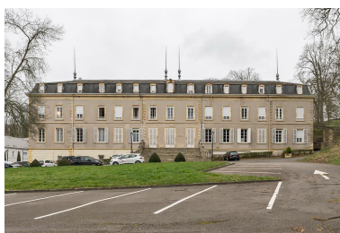
Aile nord, façade. Phot. Pierre-Marie Barbe-Richaud IVR26_20227100048NUC4A
