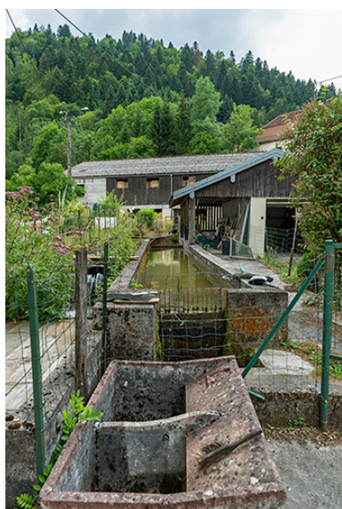
Rigole d'alimentation. Phot. Sonia Dourlot IVR43_20192500637NUC4A
