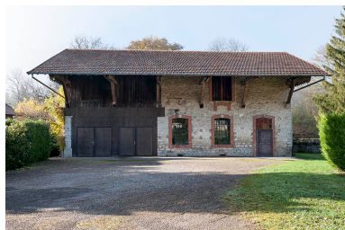
Entrepôt industriel. Face est. Phot. Jérôme Mongreville IVR43_20152502507NUC4A
