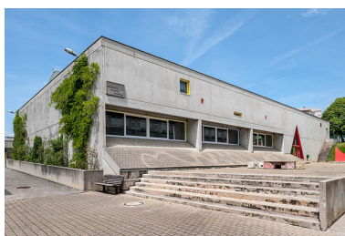
Atelier bois Phot. Jérôme Mongreville IVR43_20143900307NUC4A
