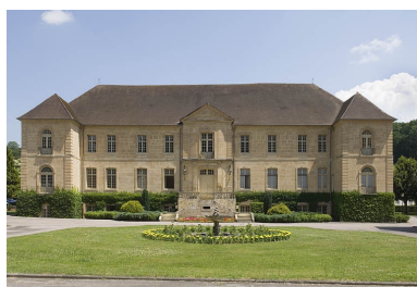
Logis abbatial. Vue de face. Phot. Jérôme Mongreville IVR43_20097000680NUC2A
