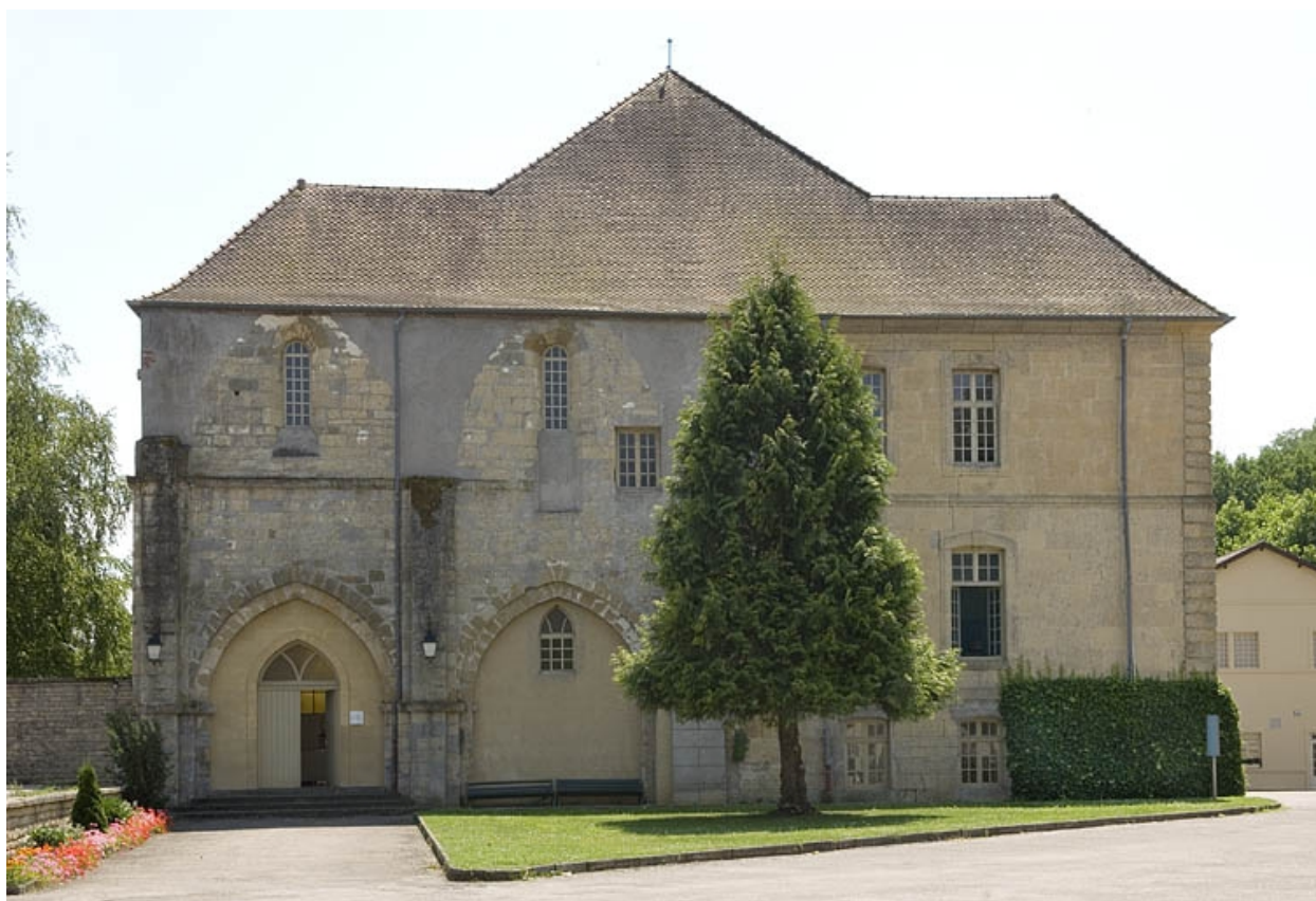
Logis abbatial. Façade nord.
