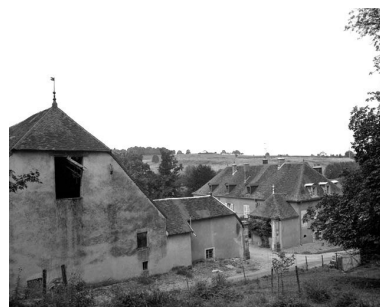
Façade principale. Phot. Yves Sancey IVR43_19843900369X
