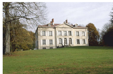
Façade ouest. Phot. Yves Sancey IVR43_20009000869ZA
