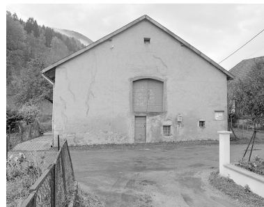
Face nord. Phot. Jérôme Mongreville IVR43_19963901640X
