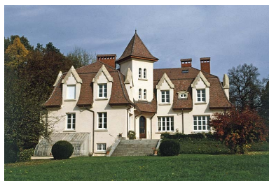
Façades ouest. Phot. Yves Sancey IVR43_20009000853ZA
