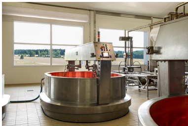
Cuve. Phot. Sonia Dourlot IVR43_20192500685NUC4A
