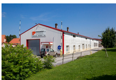
Atelier ouest. Phot. Yves Sancey IVR43_20132501408NUC2A
