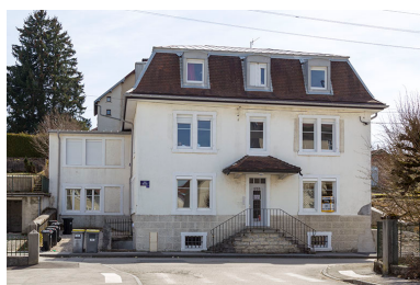
Façade antérieure. Phot. Sonia Dourlot IVR43_20152500912NUC2A
