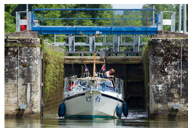
Ecluse n°43, Demangeville (70). Phot. Sonia Dourlot IVR43_20157000951NUC2A
