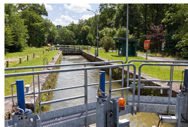
Ecluse n°40, Selles (70). Phot. Sonia Dourlot IVR43_20157000917NUC2A
