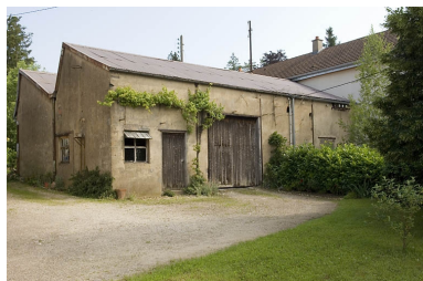
Atelier de fabrication. Phot. Jérôme Mongreville IVR43_20087000565NUC2A
