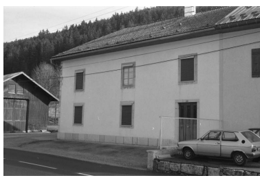
Logement patronal. Phot. Laurent Poupard IVR43_19913901613Z
