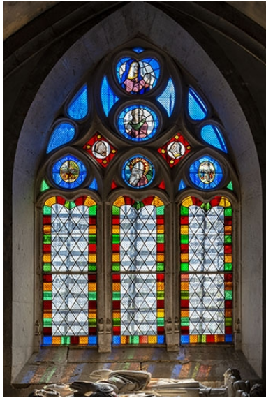
Baie 3. Phot. Jérôme Mongreville IVR43_20193900001NUC4A
