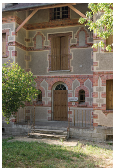
Façade principale, arrière-corps central. Phot. Pierre-Marie Barbe-Richaud IVR26_20195800507NUC4A
