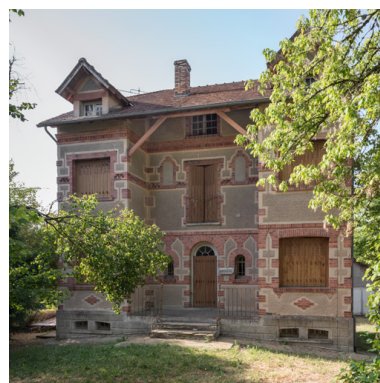
Façade principale. Phot. Pierre-Marie Barbe-Richaud IVR26_20195800508NUC2A
