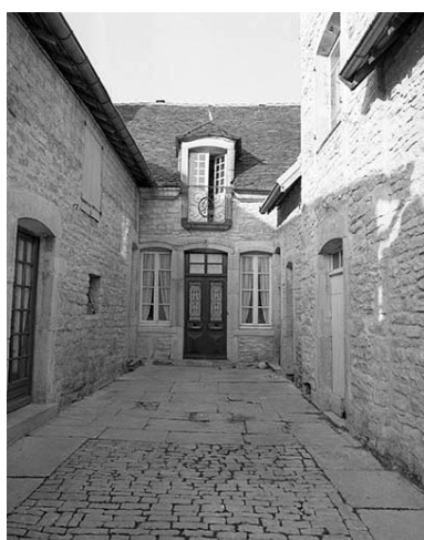
La cour. Phot. Yves Sancey IVR43_19833900052X
