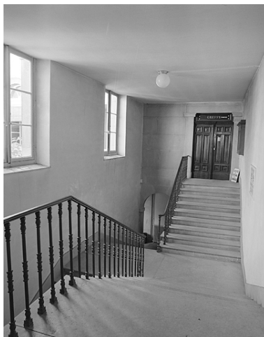
Escalier. Phot. Yves Sancey IVR43_19833900546X
