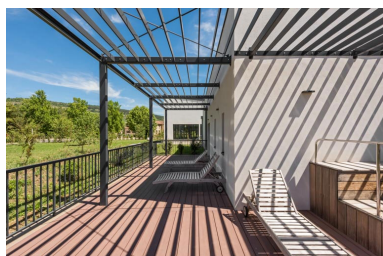
Centre thermal de 2021. Phot. Pierre-Marie Barbe-Richaud IVR26_20222100236NUC4A
