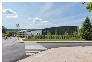
Centre thermal de 2021. Phot. Pierre-Marie Barbe-Richaud IVR26_20222100212NUC4A
