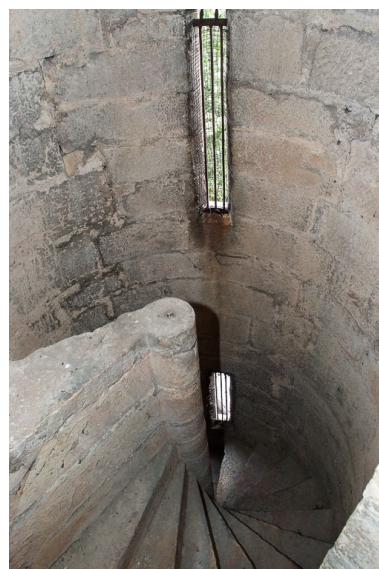
Escalier tournant. Phot. Pierre-Marie Barbe-Richaud IVR26_20152100459NUC2A
