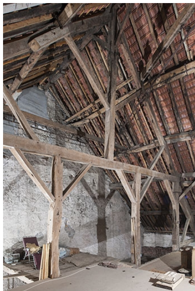
Charpente. Phot. Jérôme Mongreville IVR43_20127000447NUC4A
