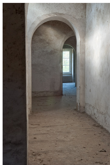
Comble : aile droite. Phot. Pierre-Marie Barbe-Richaud IVR26_20107101021NUC2A
