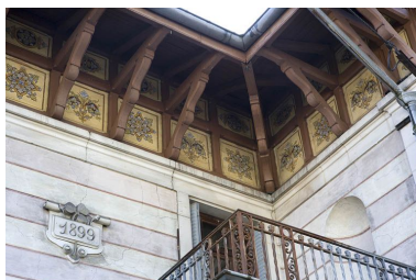
Elévation antérieure : saillie de rive. Phot. Yves Sancey IVR43_20093900167NUC2A
