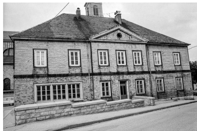
Façade antérieure. Phot. Gilbert Poinot IVR43_19752500728Z
