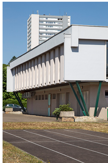
Pignon sud de la cantine. Phot. Sonia Dourlot IVR43_20147000221NUC2A
