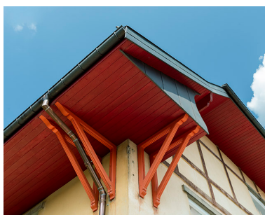
Consoles soutenant l'avant-toit. Phot. Sonia Dourlot IVR43_20192500667NUC4A
