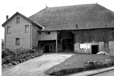
Façade postérieure. Phot. Gilbert Poinot IVR43_19752500874Z
