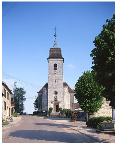
Façade antérieure. Phot. Yves Sancey IVR43_19857000073VA
