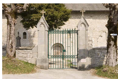
Portail. Phot. Jérôme Mongreville IVR43_20092500452NUC2A
