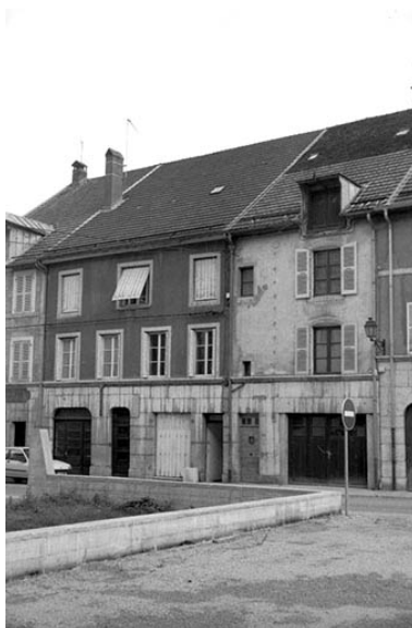
Logement patronal. Phot. Laurent Poupard IVR43_19913901307Z
