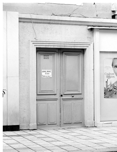
Porte principale. Phot. Yves Sancey IVR43_20033900775X
