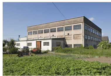
Atelier de fabrication nord. Phot. Jérôme Mongreville IVR43_20097000407NUC2A
