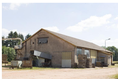
Scierie. Phot. Jérôme Mongreville IVR43_20097000424NUC2A
