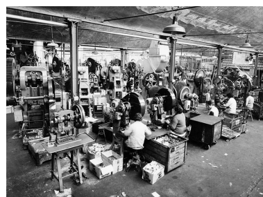
Usine Maglum. Atelier des presses. Phot. Jérôme Mongreville IVR43_20057000658NUCA
