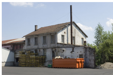
Bureaux (?). Phot. Jérôme Mongreville IVR43_20067000521NUCA
