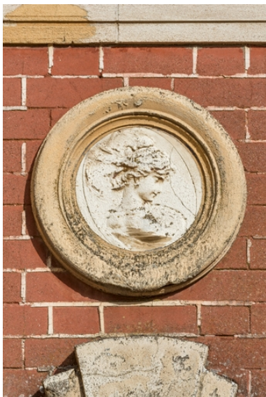
1er bas-relief. Phot. Pierre-Marie Barbe-Richaud IVR26_20222100885NUC4A
