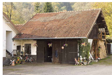
Remise. Phot. Jérôme Mongreville IVR43_20077000626NUCA
