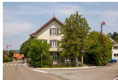
Logement patronal. Phot. Yves Sancey IVR43_20132501091NUC2A
