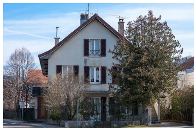
Logement patronal. Phot. Jérôme Mongreville IVR43_20142500161NUC4A
