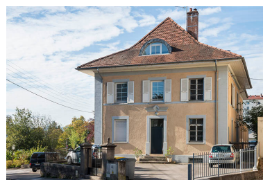
Pignon est. Phot. Jérôme Mongreville IVR43_20172501164NUC4A
