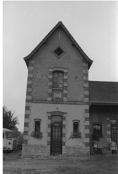
Pavillon sud, façade est. Phot. Frédéric Pillet IVR26_19997100813Z
