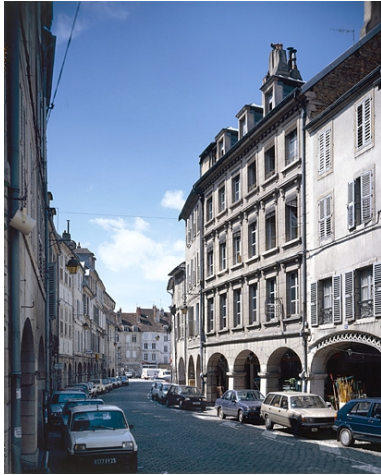
Façade antérieure. Phot. Yves Sancey IVR43_19883900110VA
