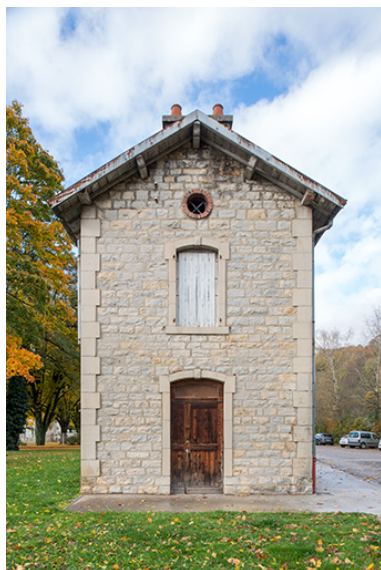
Mur-pignon sud. Phot. Nicolas Waltefaugle IVR43_20253900351NUC4A
