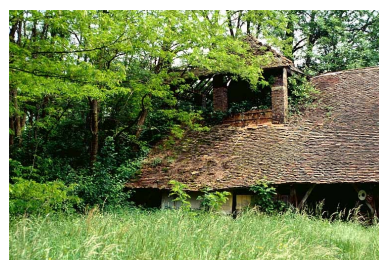
Four industriel. Phot. Jérôme Mongreville IVR43_19963900503ZA
