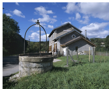
Puits. Phot. Yves Sancey IVR43_20043900454XA
