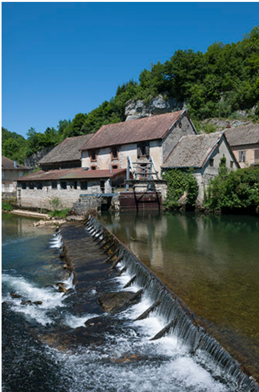
Atelier Auguste Louvrier, Lods.
