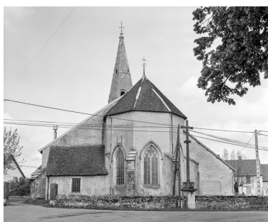
Abside. Phot. Yves Sancey IVR43_19773900220X
