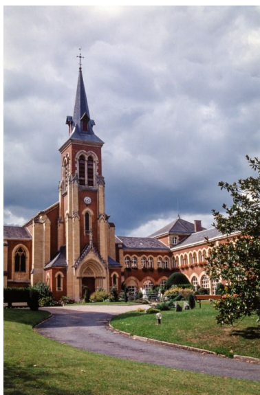
Chapelle. Phot. Jean-Luc Duthu IVR26_20017100700ZA
