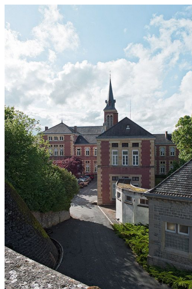
Elévation sud-est. Phot. Pierre-Marie Barbe-Richaud IVR26_20107100779NUC2A
