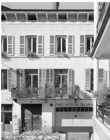
Elévation antérieure. Phot. Yves Sancey IVR43_20033900680X
