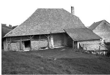
Façade postérieure. Phot. Gilbert Poinot IVR43_19762500946Z
